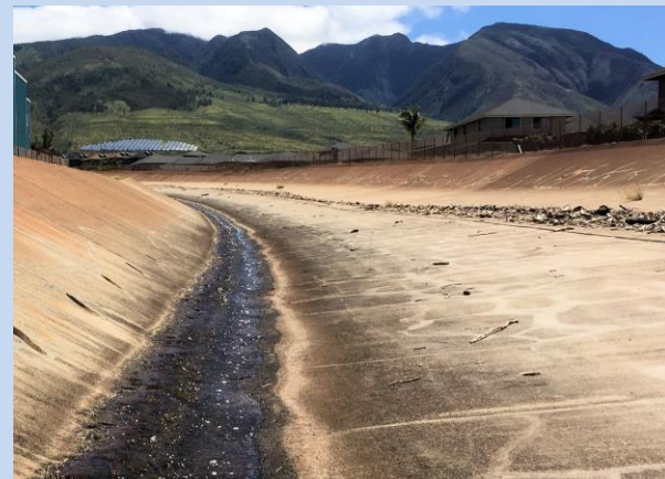
Stable concrete-lined stream channel at Kahoma Stream, Lahaina, Maui
